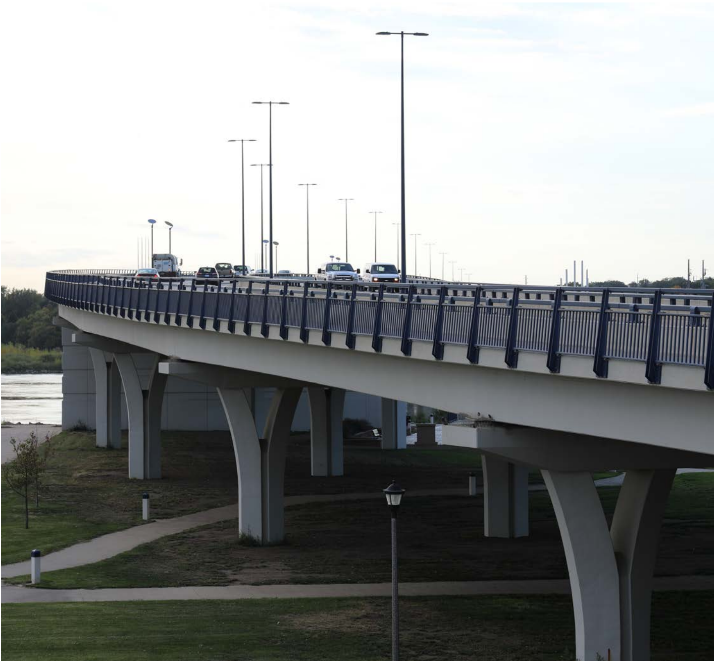
Figure 4.12: Memorial Bridge Over the Missouri River
